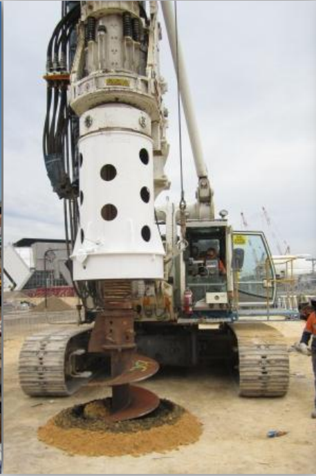
Bored Pile Set Up
